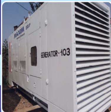
Generator; Brand: Himonsa; Capacity: 50 KVA
