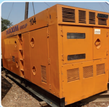
Generator; Brand: Himonsa; Capacity: 50 KVA
