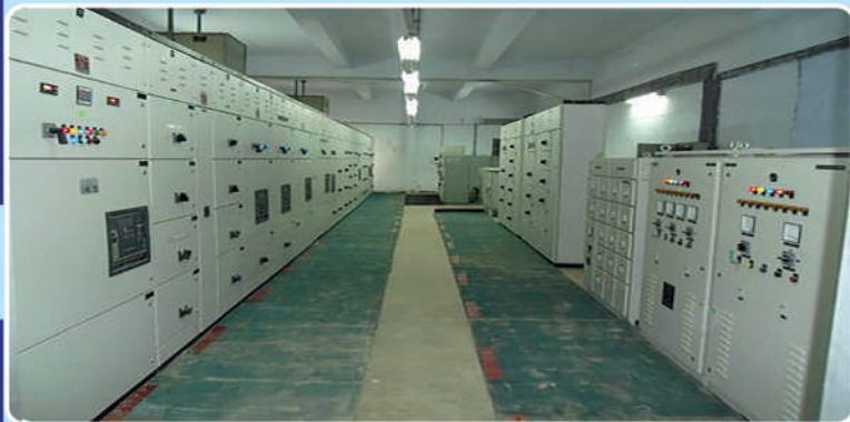
Panel Fixing & Cable Termination Work
